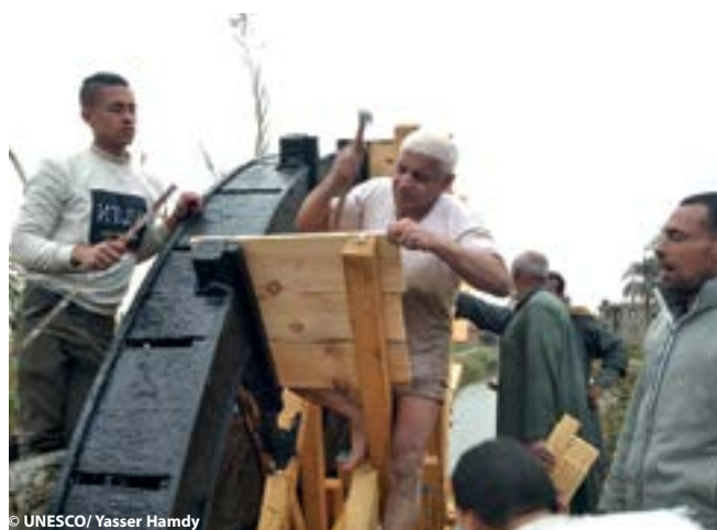
Image 24: Installing the waterwheel
